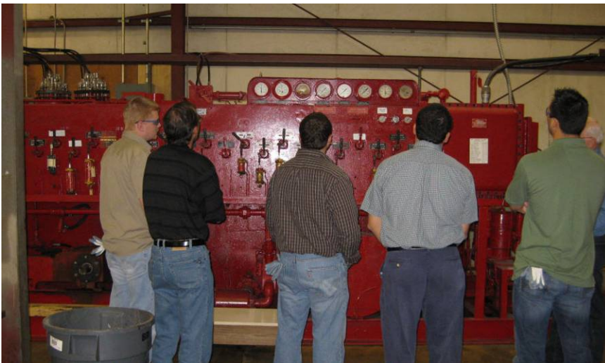
Students reviewing subsea control unit
