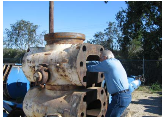
Instructor Ray Marek demonstrates a baseline ram cavity inspection on a ram BOP
