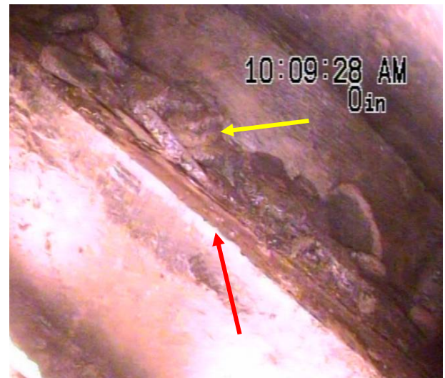
Figure 4: Debris on the blind shear lower blade.
